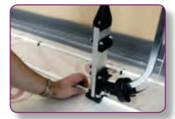
**STEP 4.** Using the staple gun, fix the pipework to the installation in the desired pattern (see page 15 images on patterns of pipework). Starting the first circuit 75mm from the perimeter and staples should be approximately 500mm apart. More staples maybe needed on bends.
