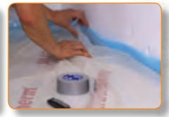
**STEP 3.** BS EN 1264 Part 4 requires a protective membrane placed over the insulation layer and it specifies Polyethylene film of at least 0.15mm thickness with 80mm overlaps or a similar product which performs the same function e.g. Aluminium Foil fitted at the factory.
