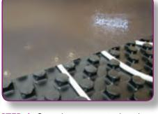
**STEP 6.** Once the pipe circuits have been installed and pressure tested, the system should remain under pressure (6 bar) in order to prevent the risk of any damage being caused to the pipe while the screed is being applied. When applying the screed cover, care should be taken to ensure that the screed is tightly compacted.
