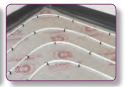
**STEP 6.** Once the pipe circuit has been installed and pressure tested, the system should remain under pressure (6 bar) in order to help prevent the risk of any damage to the pipe while the screed is being applied. When applying the screed, care should be taken to ensure the screed is tightly compacted around the pipe ensuring no voids are present.
