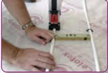
**STEP 5.** When using the pipe, unroll it from the outside of the coil and do not try to uncoil it from the centre, this will make the process easier. Keeping the first run of pipe around the perimeter straight and using a gauge to keep the designed pipe centres even will also help the installation process.
