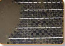
**STEP 5.** Screed is placed on top of the pipe circuits.
