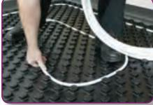
**STEP 5.** Starting from a manifold, after establishing the area to be covered, unroll the pipe and push firmly into the gap between the egg box sections. Cover the designed area in the appropriate pattern and return the pipework to the manifold.
