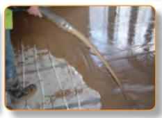
**STEP 6.** Screed depths need to be taken into consideration as part of the floor build thickness. (See page 20 for typical floor section).
