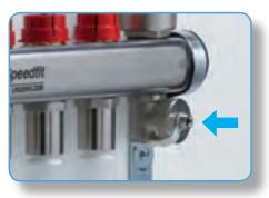
**STEP 5.** Connect the fill hose to the top hose connector valve on the manifold Flow Rail. Ensure the valve is in the open position.
