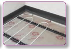
**STEP 6.** A serpentine pattern is usually the most convenient to use with the mounting rail system. Ensure to allow enough space at the end of the circuits for the flow and return from the manifolds.
