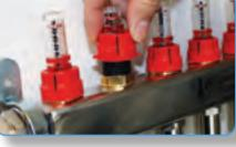
STEP 2. Open all flow gauges at the top of the manifold by lifting the locking cover and turning the adjuster anti-clockwise.
