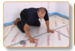
**STEP 4.** This vapour barrier will prevent the contamination of the insulation by the screed. It will also prevent liquid type screeds from flowing between gaps in the insulation and "floating" the boards during installation.
