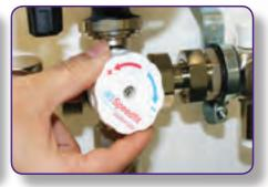
**STEP 6.** The designed temperature through the circuits is controlled by turning the blending valve knob to the desired temperature.
