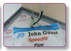
**STEP 3.** After establishing the area to be covered by the pipe circuit, connect to the manifold and start the circuit. If the circuit has to pass through other heated zones before reaching the zone it is intended to heat, conduit may be required.
