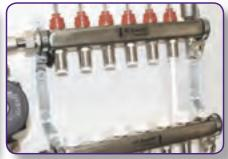
**STEP 3.** Connect the pipework to the manifold following the guidelines for fitting JG pipe and fitting. It is best to start from one end of the manifold and work to the other. The use of JG conduit elbows will make the process easier and neater and enable the conduit to be inserted into the socket end.
