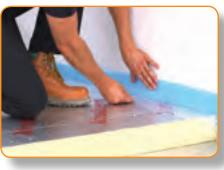
**STEP 2.** An expansion strip is required to accommodate the expansion which will occur within the screed as the result of it heating up. This expansion strip should be fitted round the perimeter of the room and taped to the membrane.
