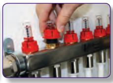
**STEP 5.** The flow meters at the top of the manifold give a visual indication of the amount of water flowing through each circuit. The amount of flow will depend on the length of circuit and the temperature drop required. Generally the shorter the circuit the more restriction will be needed; this is called balancing the system.
