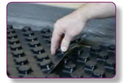
**STEP 4.** When a pumped (liquid) screed is to be used it is essential that all of the panel joints are made correctly and that no panels are allowed to simply 'butt-up' as this may allow the screed to flow below the panels causing them to rise up.
