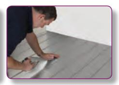
**STEP 3.** After placing the boards and ensuring they are flat and level and the joints are butted up firmly. Tape the joints using JGTAPE.
