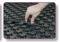
**STEP 3.** The "egg box" sections of the panel clip firmly together to make a continuous seal. Floor panels should not be used at the base of a manifold as pipes need to be closer together than the floor panels will allow. Pipes around this area should be secured using pipe staples.
