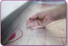
**STEP 2.** An expansion strip is required around the perimeter of the room to accommodate the expansion which will occur within the screed as a result of heating up. This should be fitted around the perimeter of the room and taped to the membrane.
