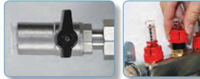
STEP 1. Turn off any electrical equipment. Isolate the manifold from the heating system by turning the ball valves to the off position.
